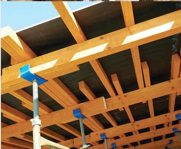
WOOD LINE LVL is used for the construction with high load bearing such as beams, pillars, flooring structures...
